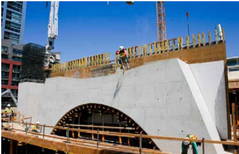
Photos: Morley Construction
